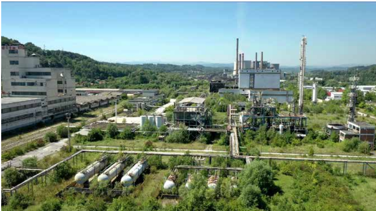
Corroding pipes in HAK factory with unknown quantities of chlorine.
